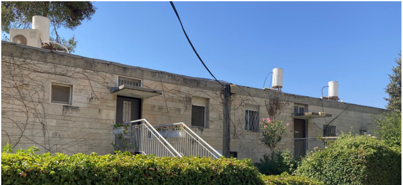
Figure 2: Adjacent Houses in the Neve Sha'anun Neighborhood
